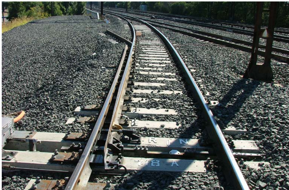
Figure 4 – Example of catchpoint with good landing zone
